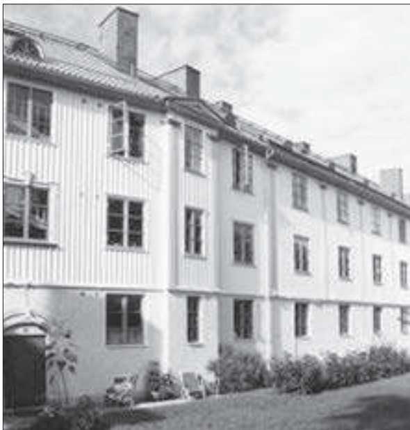
Kv 4 Kynnefjäll. Gårdsfasad, kv 4:17–19.
